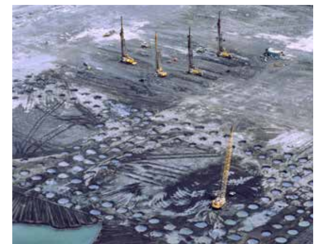
Around the clock ground improvement to consolidate the foundation
