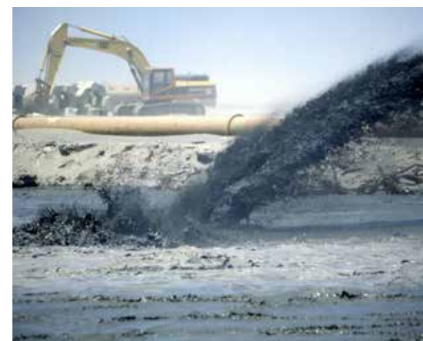
Pumping sand to fill the sea
